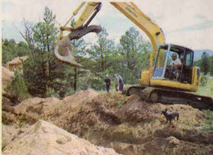
Excavating the site for a geothermal system. Courtesy photo.
